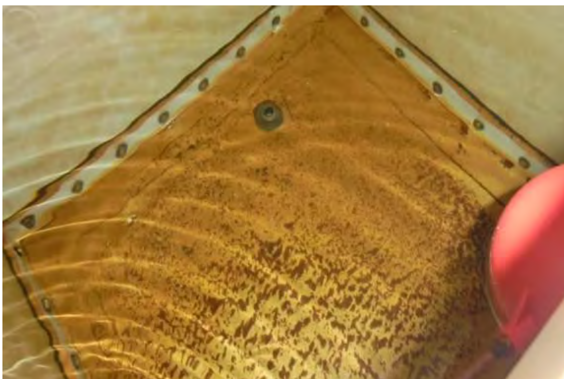
CWS Tank No. 1 – Light Sedimental Accumulations
