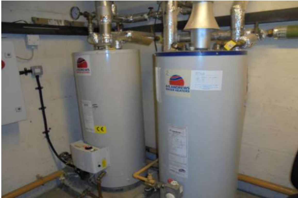
Gas Fired Water Heaters – General Arrangement
