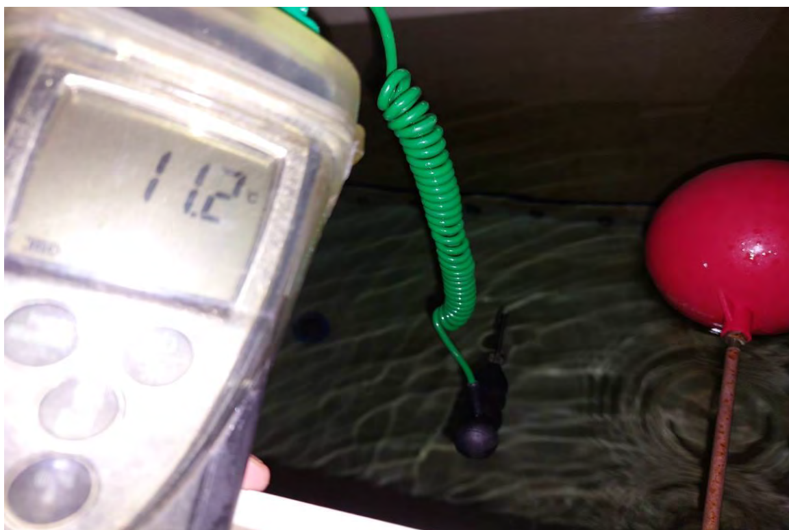
CWS Tank No.1 – Contents Temperature 11.2°C
