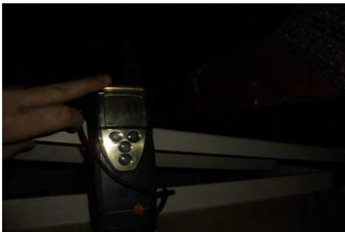
CWS Tank No. 1 – Contents Temperature Satisfactory
