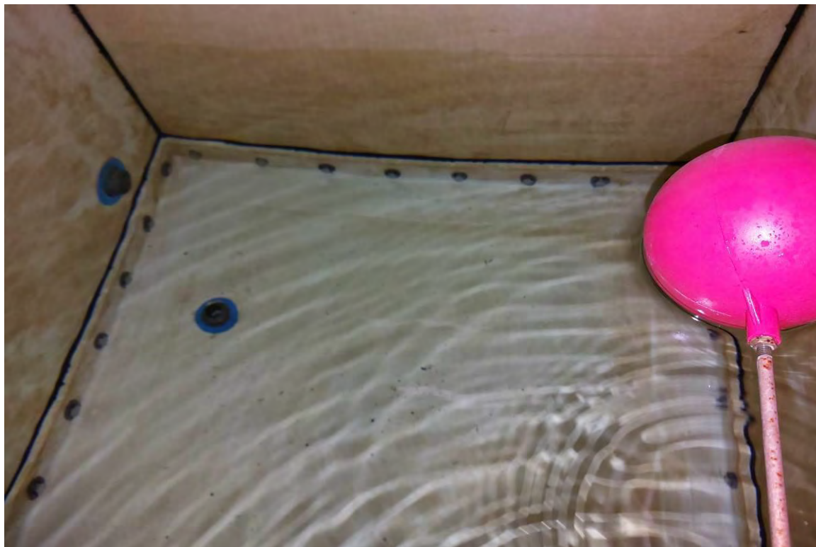
CWS Tank No.1 – Acceptable Condition with Moderate Sediment at Base
