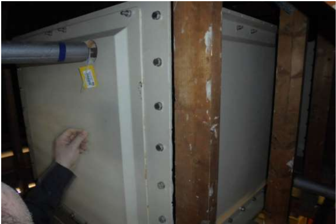
Roofspace CWS Tank – Pre-Insulated Sectional Construction
