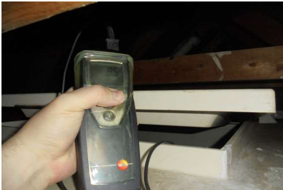
CWS Tank No. 1 – Contents Temperature at 9.5°C
