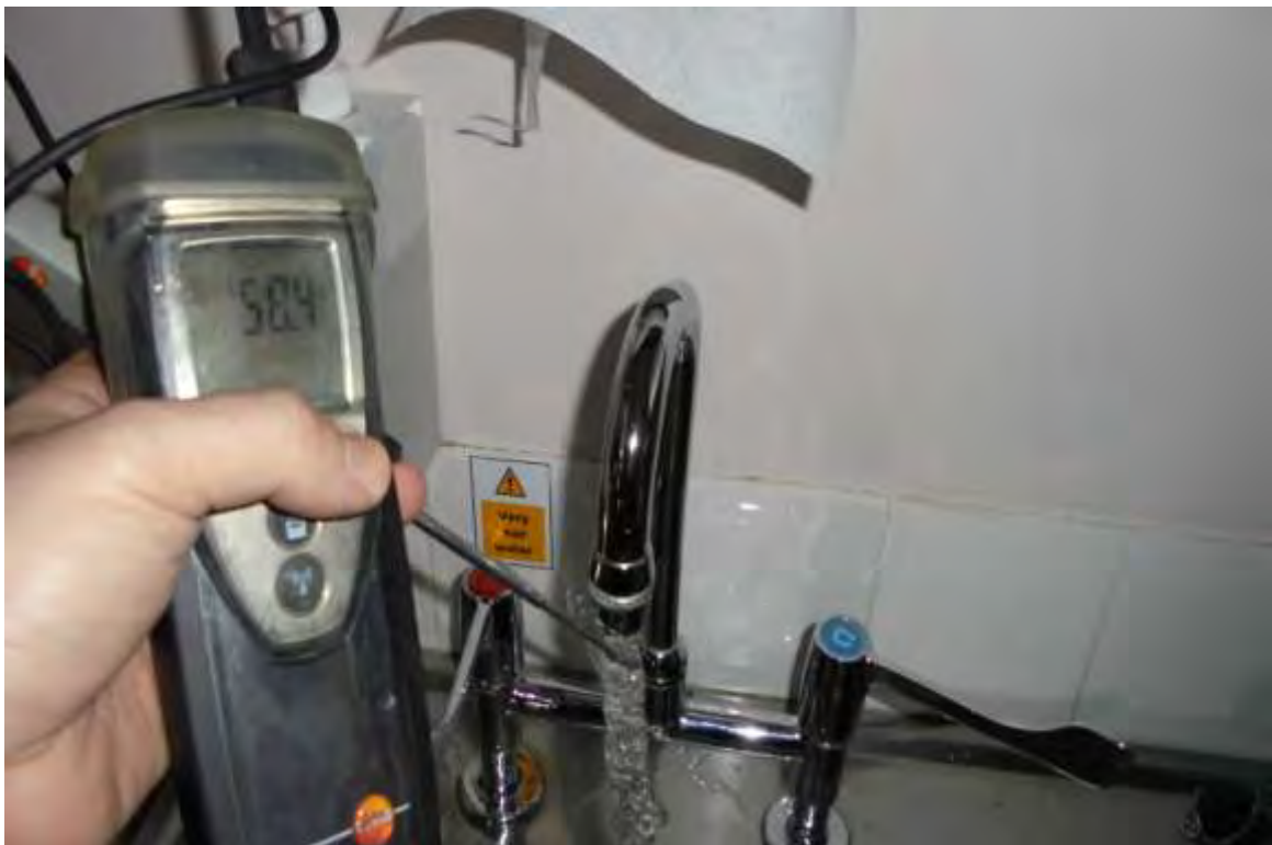
Treatment Room G/49 Sink – Hot Water Satisfactory After Extended Flush
