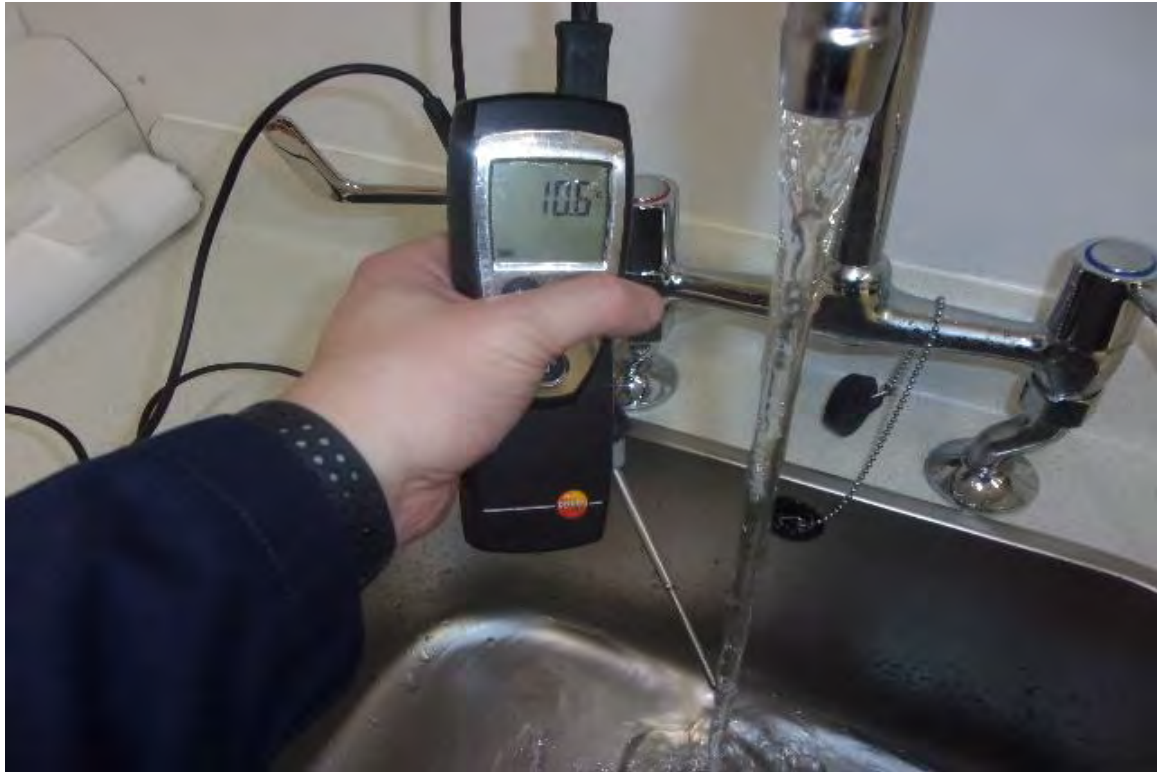
Consultant Room 1 (G/55) Sink - Cold Water Outlet Temperature Satisfactory
