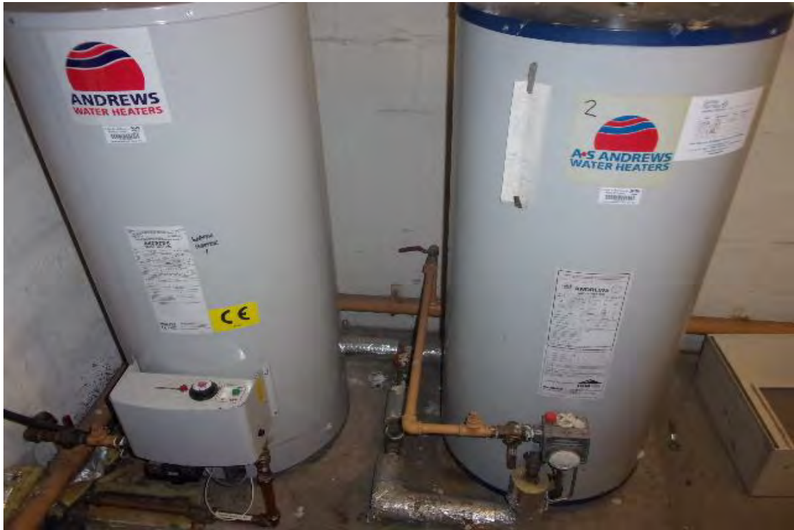
Plantroom Gas Fired Water Heaters – General Arrangement
