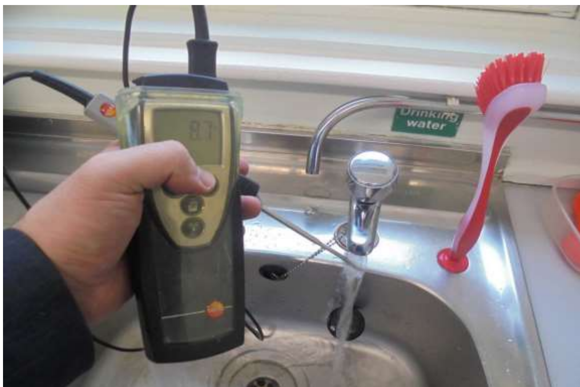
1 st Floor Staff Room Kitchen Sink - Cold Water Outlet Temperature Satisfactory
