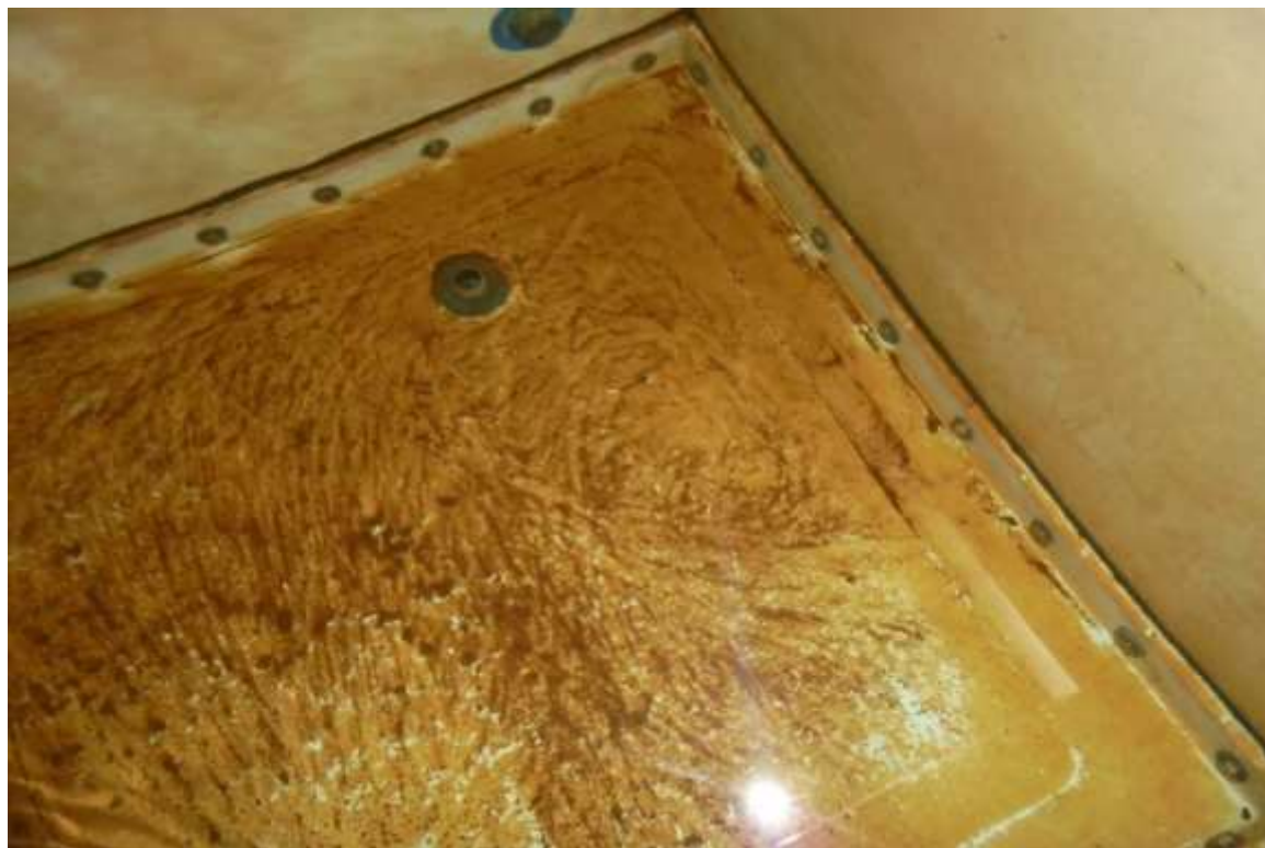
CWS Tank No. 1 – Light Sedimental Accumulations
