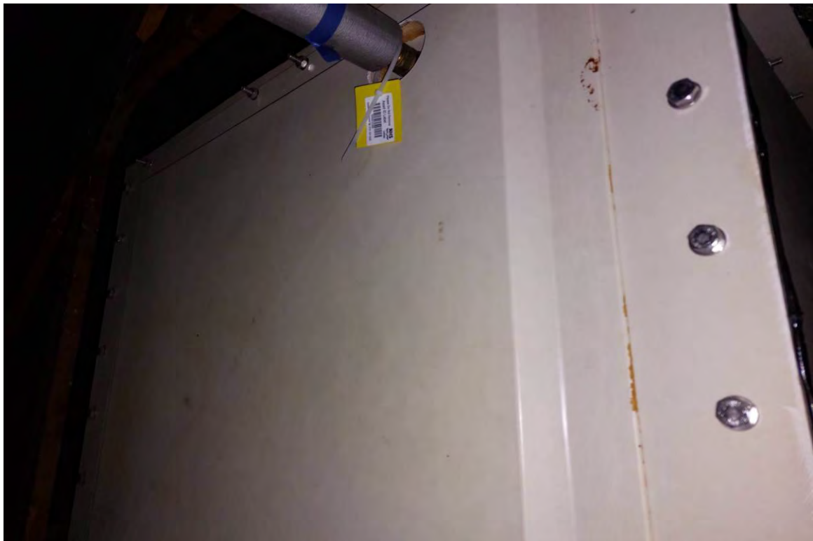
Roofspace CWS Tank – Pre-Insulated Sectional Construction
