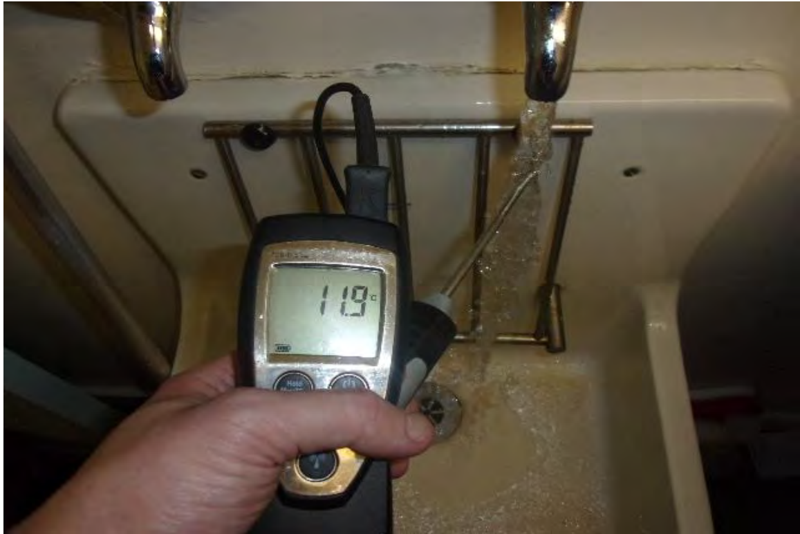
Cleaners Cupboard (G/49) Sink – Cold Water Outlet Temperature Satisfactory
