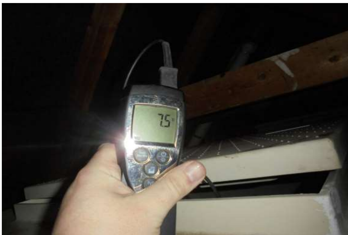
CWS Tank No.1 – Contents Temperature 7.5°C
