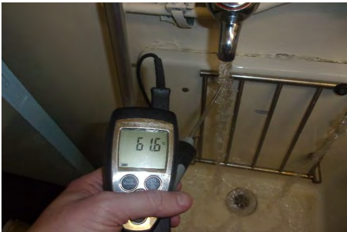
Cleaners Cupboard (G/49) Sink – Hot Water Outlet Temperature Satisfactory
