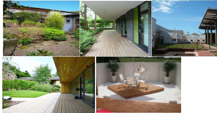
(from top left) Glasgow Homoeopathic Hospital; Kentish Town Health Centre; The Bamburgh Clinic; Firrhill Respice Centre.
