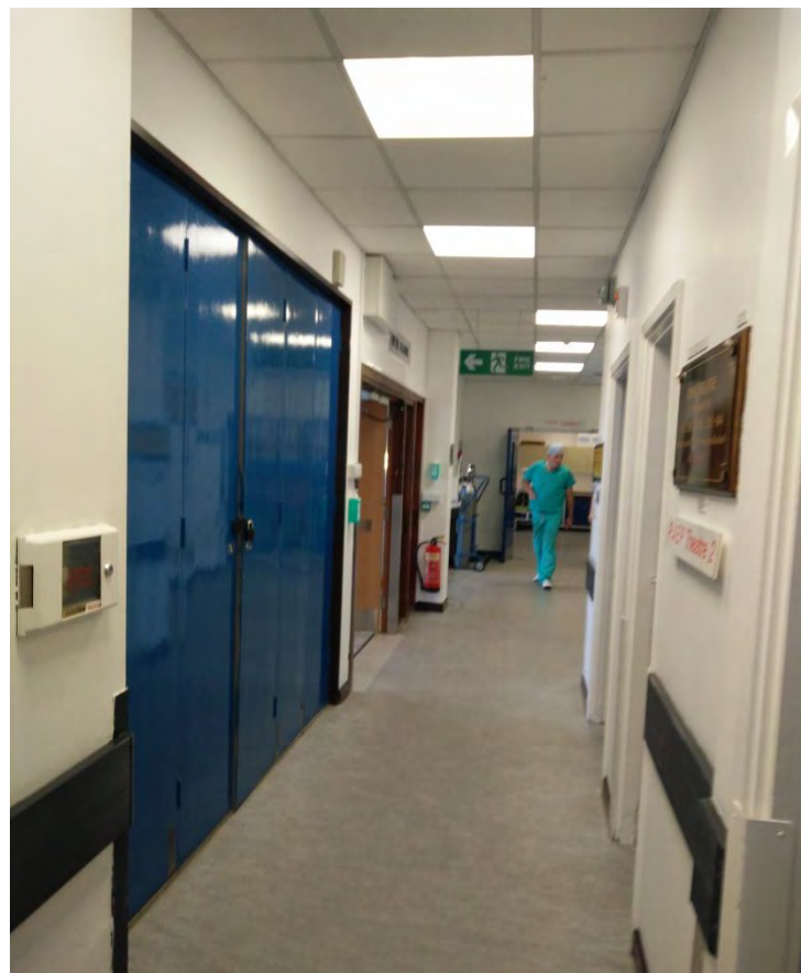
Figure 10 - Along the narrow theatre corridor, passing the main electrical switch cupboard, back to the lift on the stairwell
